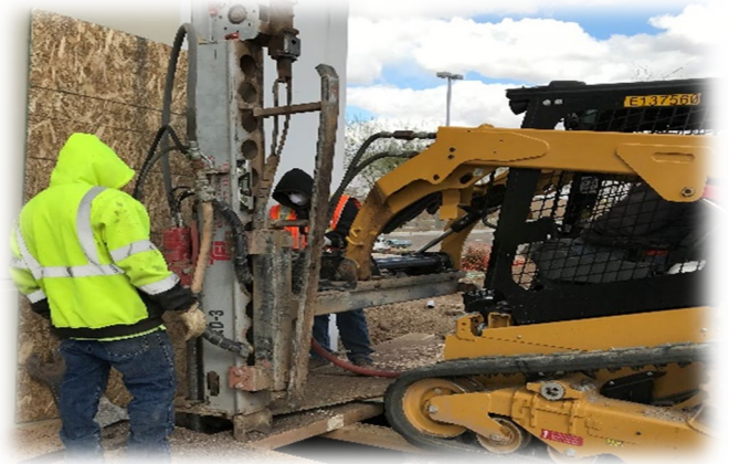
Down in the hole pre-drilling
