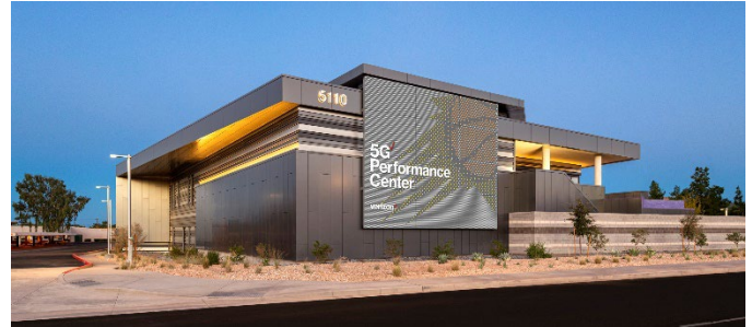
Exterior of Phoenix Suns Verizon 5G Performance Center
