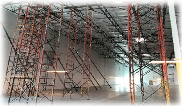
Emergency shoring of roof and tilt walls
