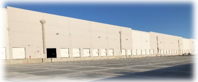
Project at completion
