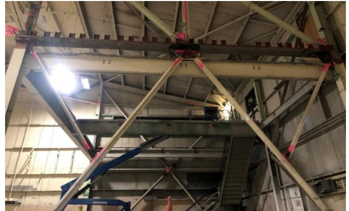
Double Angle Braces that had to be Removed and Replaced
