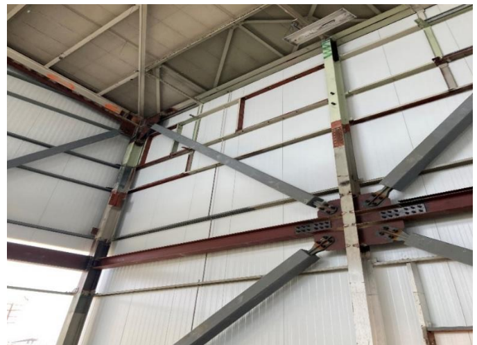
New Buckling Restrained Braces (BRB'S) in Place
