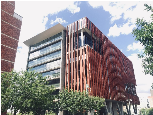
HSIB Elevation – forum area and ‘V’ columns at ground level
