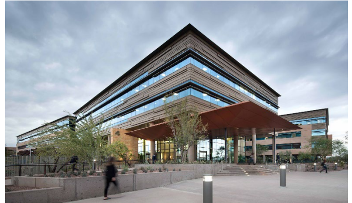
Exterior View of American Express Canyon Office Building
