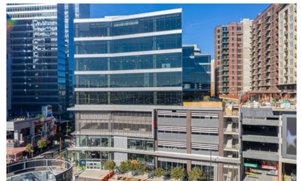
Block 23, 5 th level Amenity Deck
